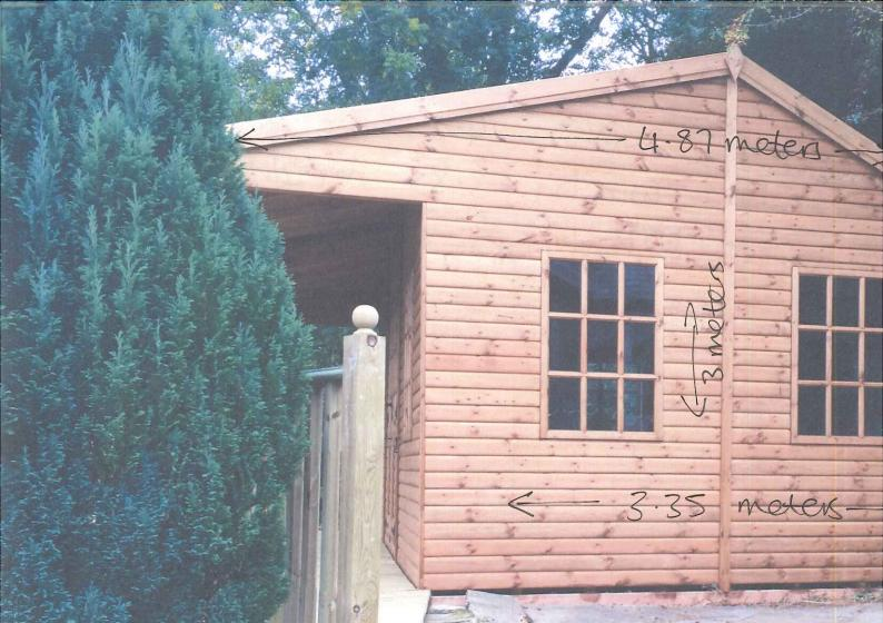
Roof width 4.87 meters NYMANDA Shed width 3.35 meters 23 JUN 2015 Shed height 3 meters
