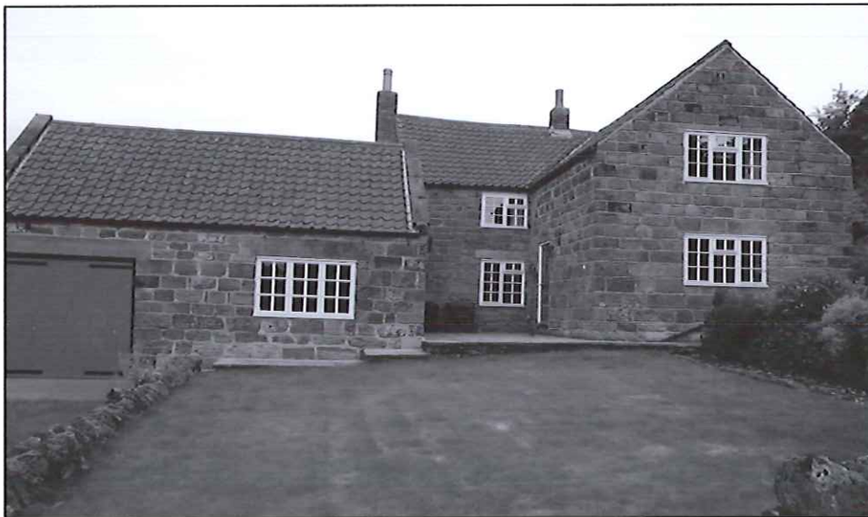
Figure 9: Front (west side) of house
