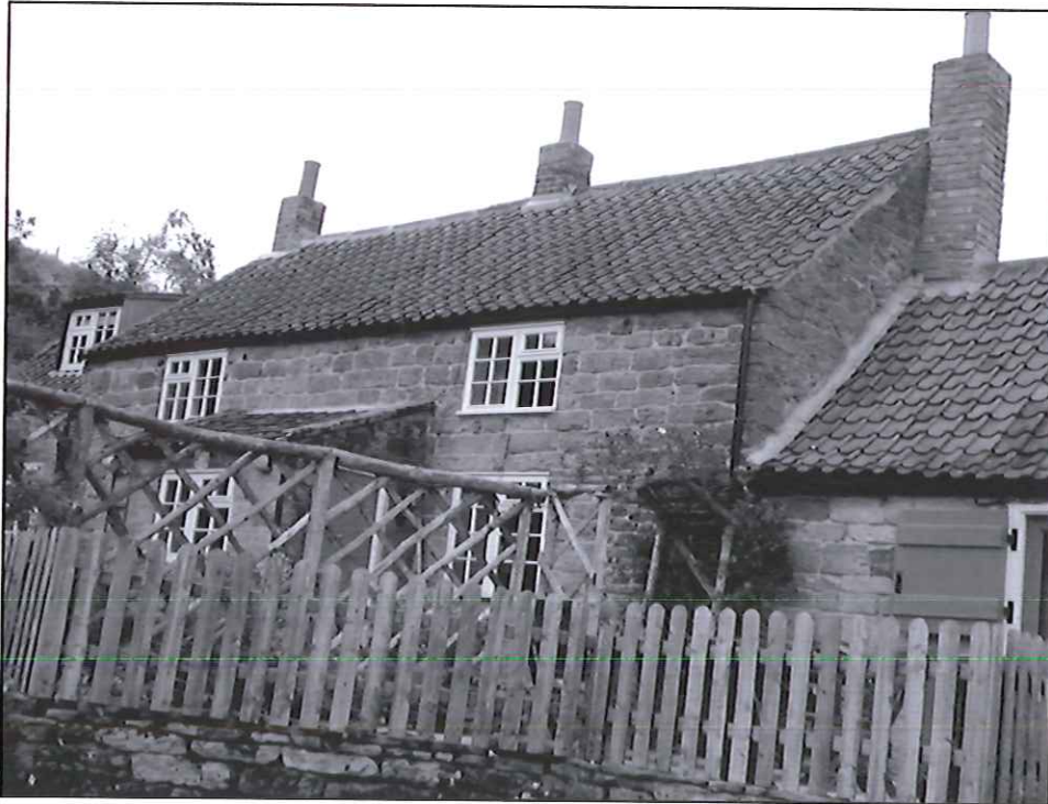
Figure 10: Rear (east side) of house, south end
