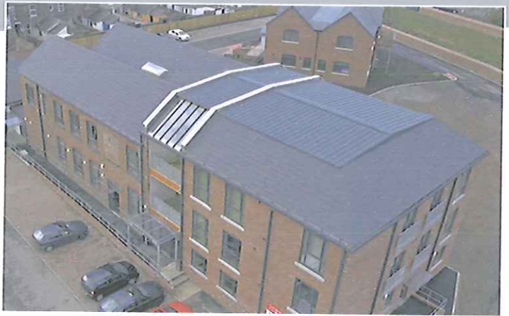
Above: Telford House, Riverside View, Carlisle. Meta-SlatePlus roofing system to a conversion of an existing building.
