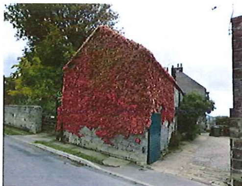
Photo 2: Northern gable end is covered in ivy making it difficult to identify crevices
