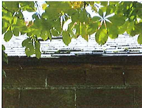
Photo 10: Eaves are obscured by guttering. Shallow masonry crevices in east wall
