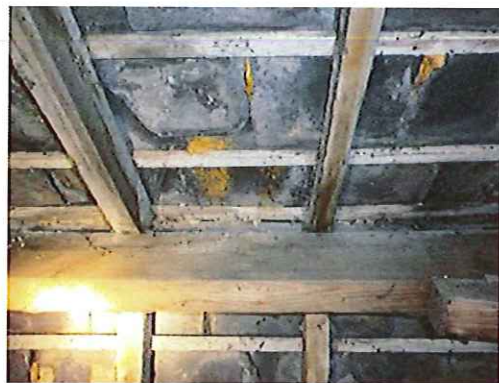
Photo 4: Internal ridge of store room 1
