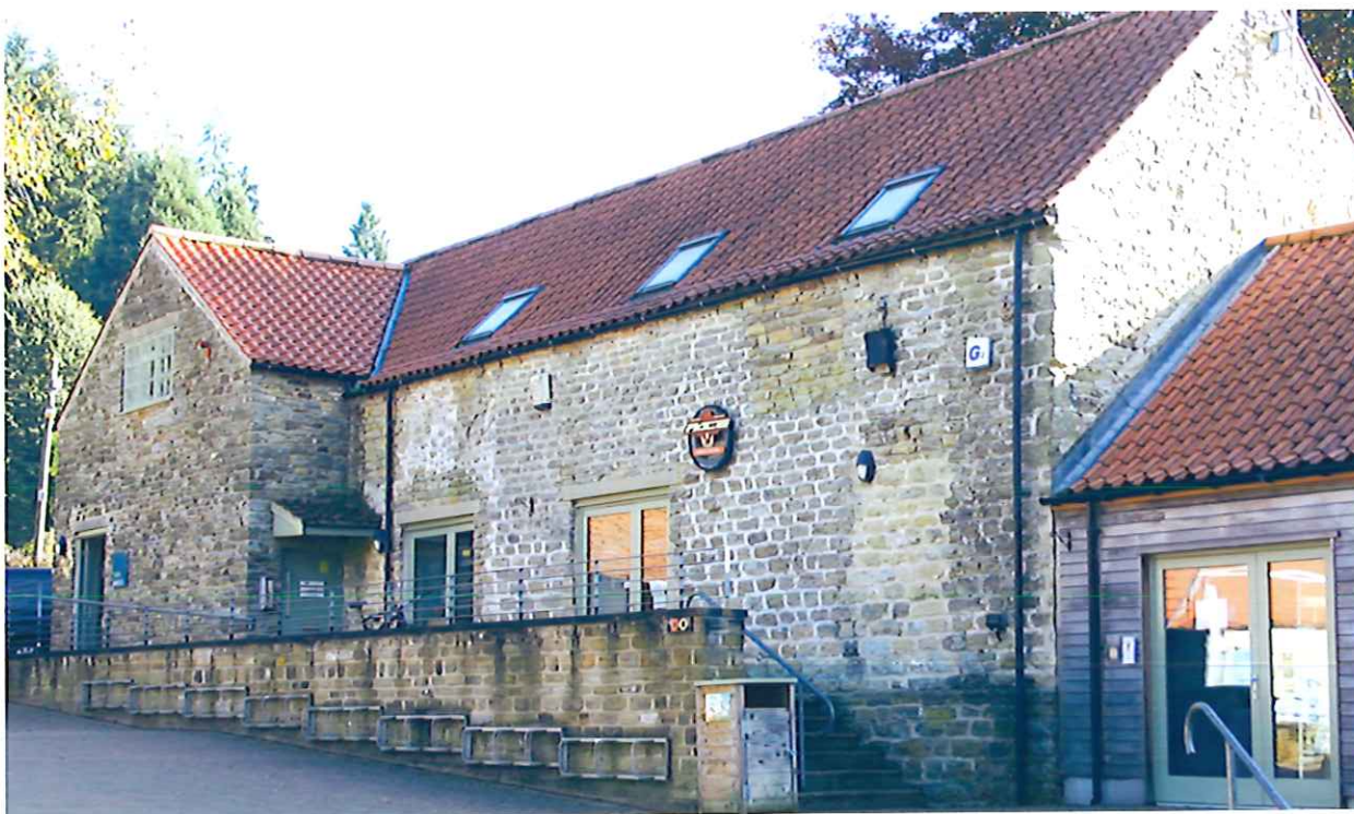
Building adjacent the Bike Barn (north elevation)
