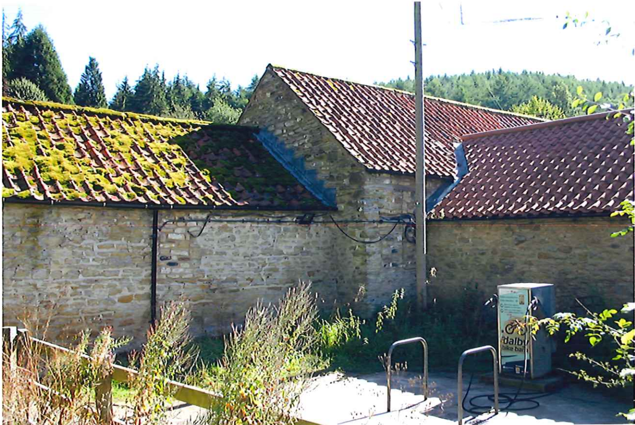
Part rear elevation (west)
