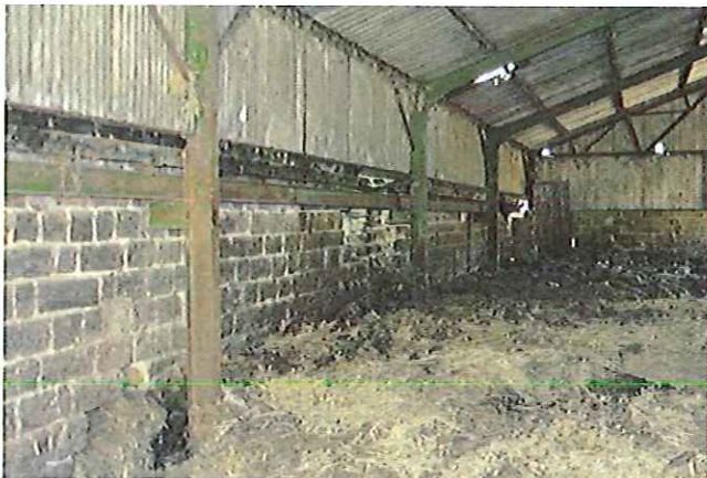
Photo 12: Rear wall of stable block.
