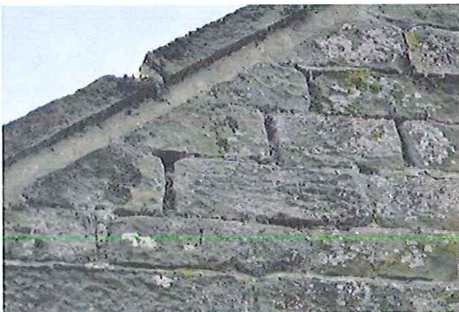
Photo 8 and 9: Cracks and holes in gable end wall.
