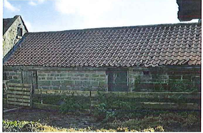
Photo 24: Rear Wall of adjoining stores.
