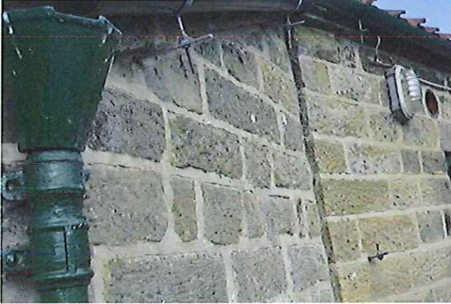
Photo 23: Walls and guttering
