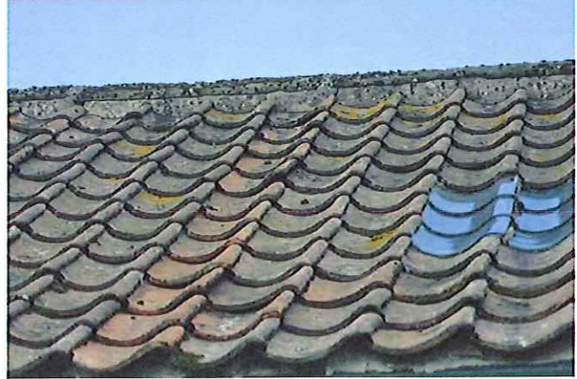
Photos 4 and 5: Photos of roof showing some raised and broken tiles, but intact ridge tiles and pointing.
