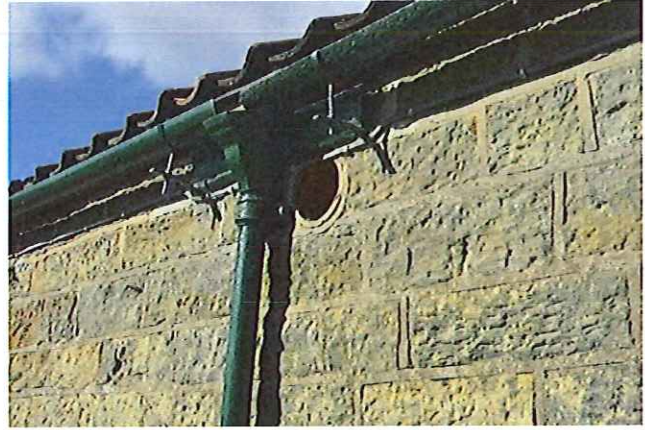
Photo 7: Ventilation holes
