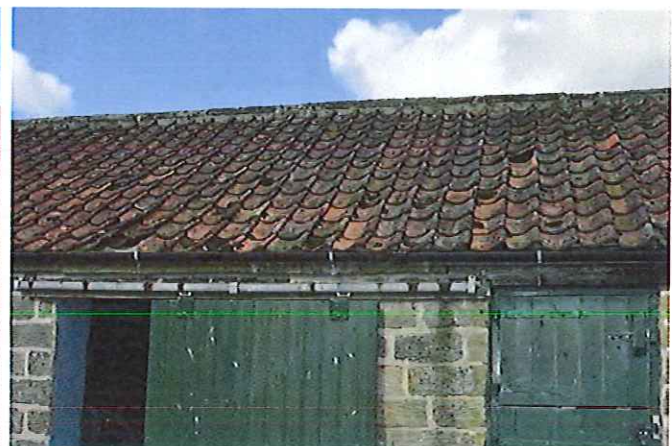
Photo 22: Roof of adjoining stores
