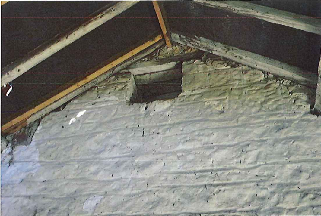
Photo 14: Opening through internal wall
