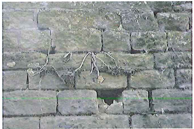
Photo 7: Ventilation holes
