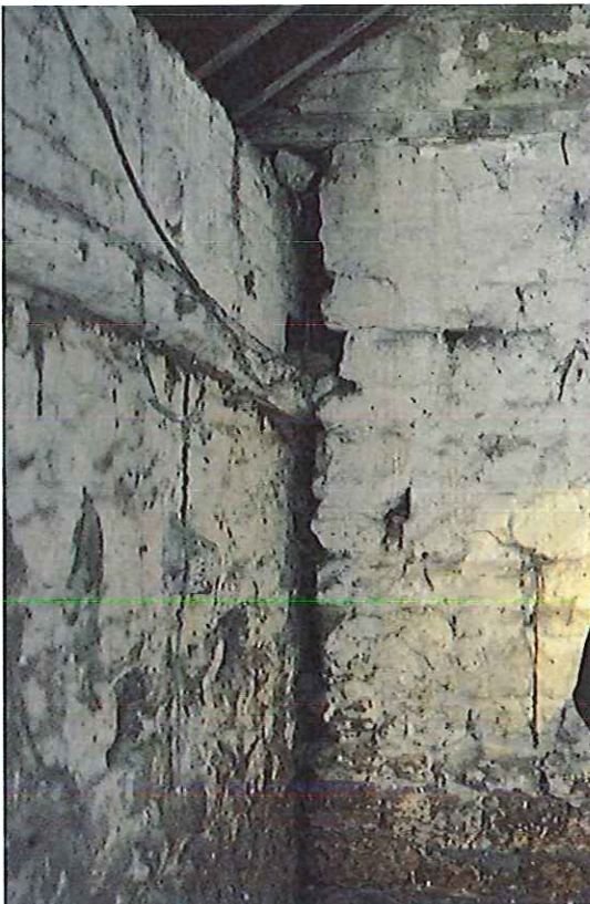
Photo 15 and 16: Cracks between internal and external walls.
