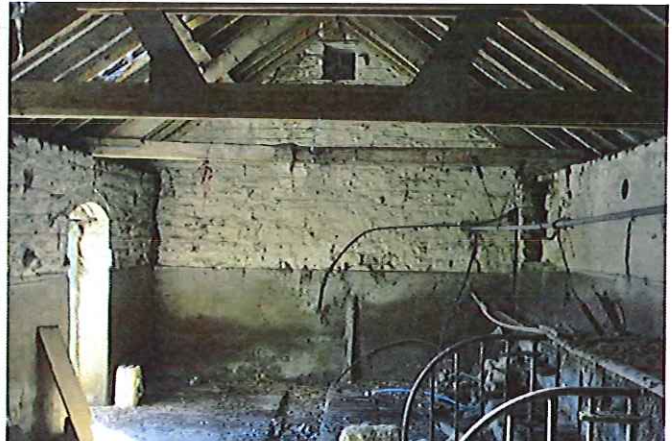
Photo 20: Interior of main area.
