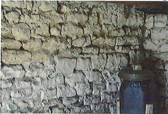
Photo 27: 3 rd store room.
