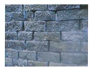
Plate 4 Mortar Loss to Gable
