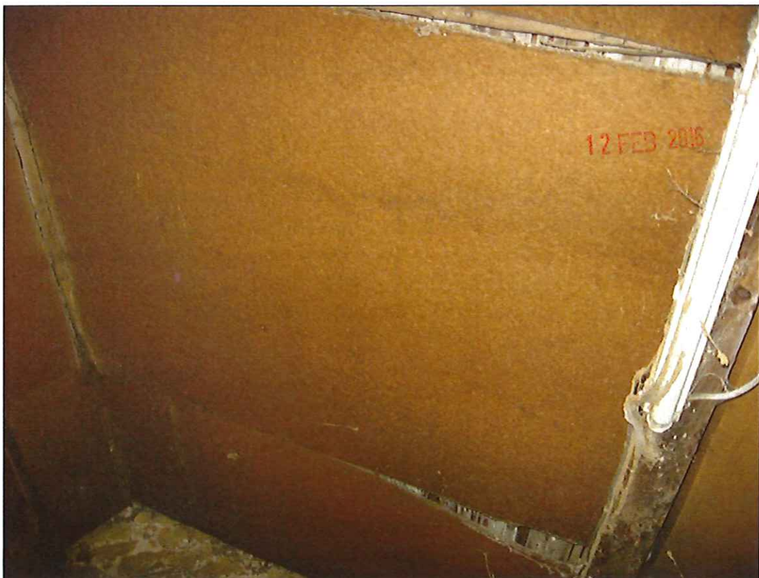
Figure 10: Underside of roof
