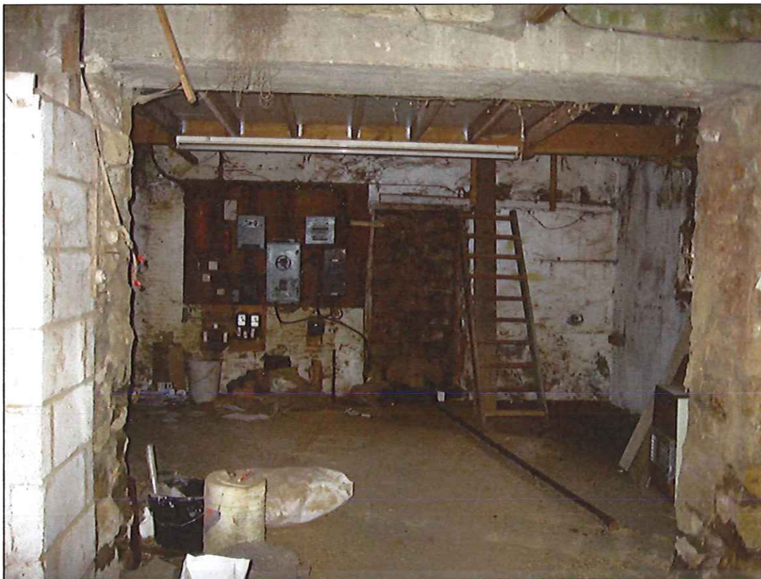
Figure 9: Interior of roadside building
