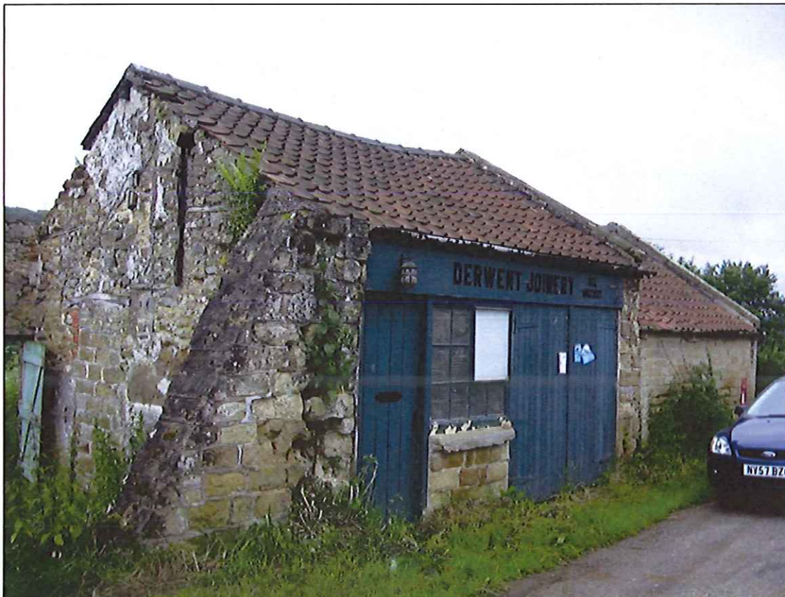
Figure 6: Roadside building, west side
