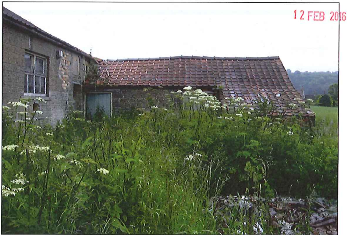
Figure 8: Rear building, south side
