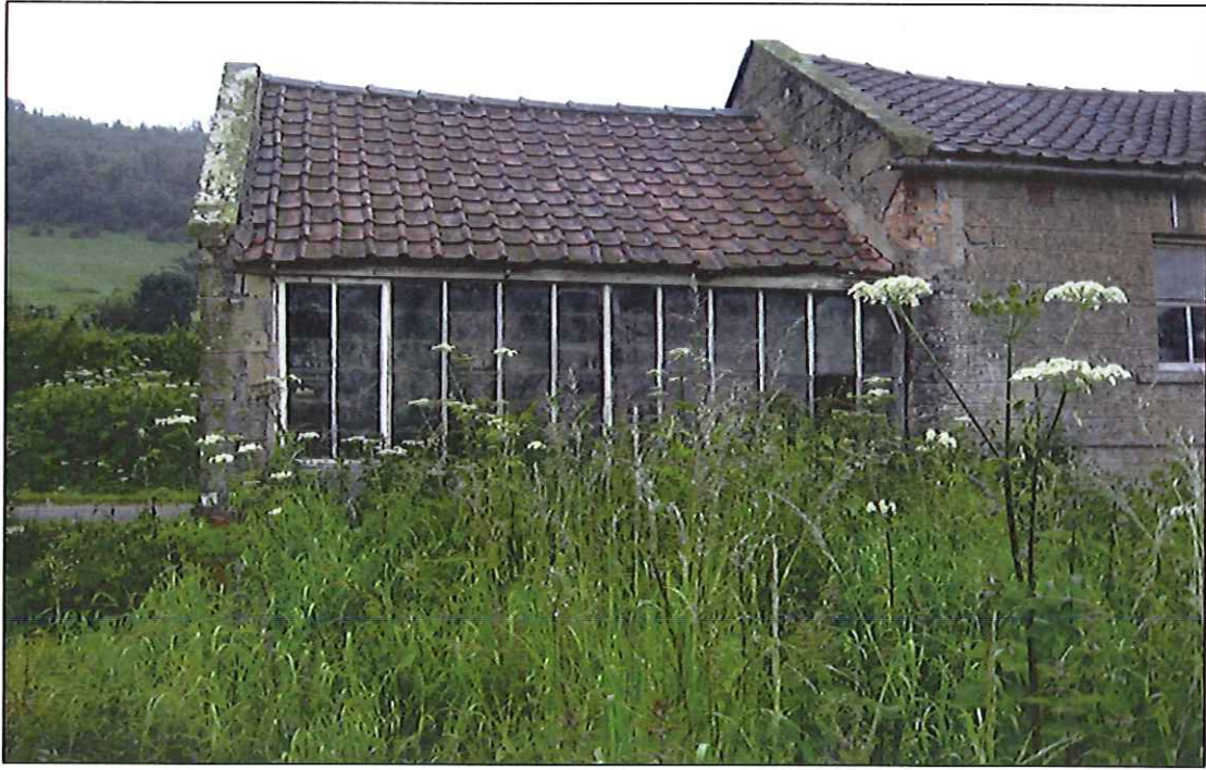
Figure 7: Roadside building, east side, south end
