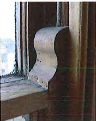
Details of the existing central dormer window
