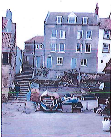
1990's photo taken around the time of the sale of the property by Leeds University to Jean Mellalieu
