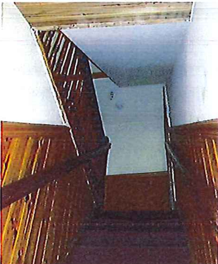
Existing Central Staircase
