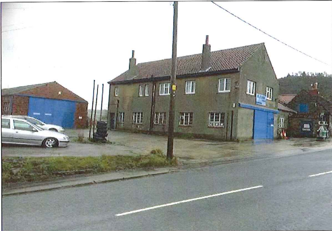
Photograph 1 Blue Bank Garage
