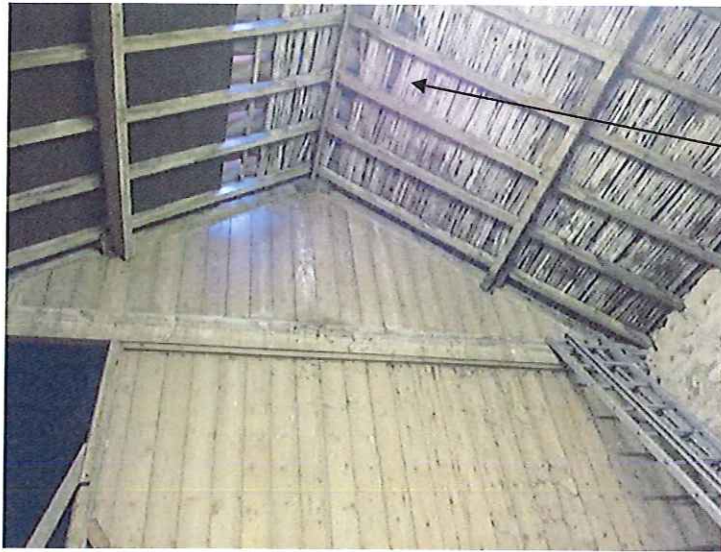
Plate 2 –Internal roof structure
