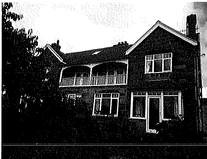
Western façade of 4 Echo Hill facing Sleights village
